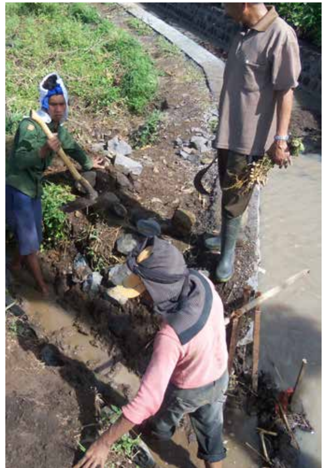
Village Secretary overseeing the construction of the the new drainage system
