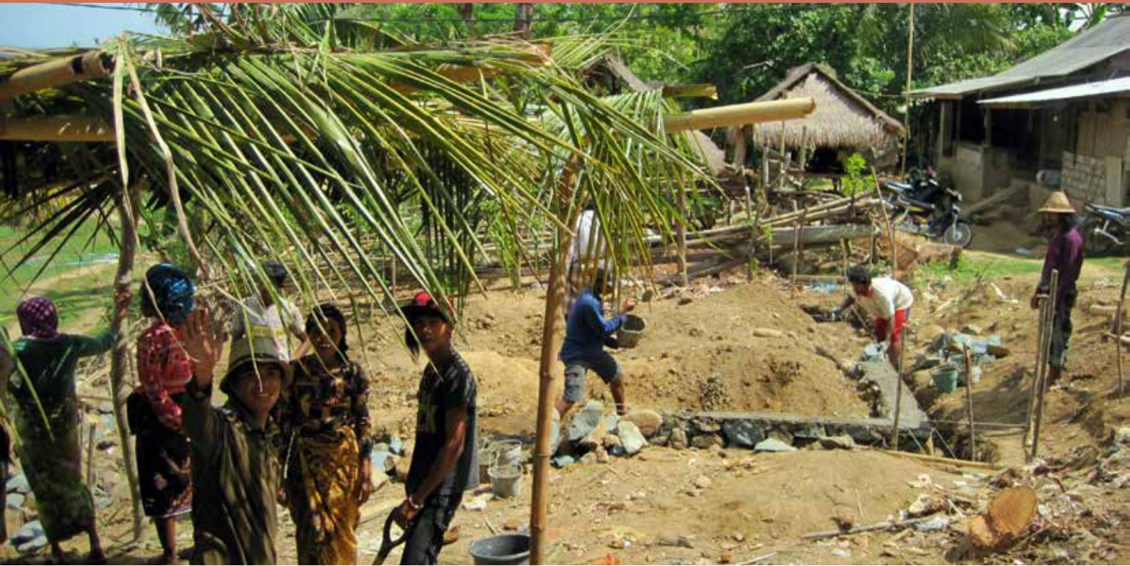
● Community participation in gotong royong to build the mushola - NTB
