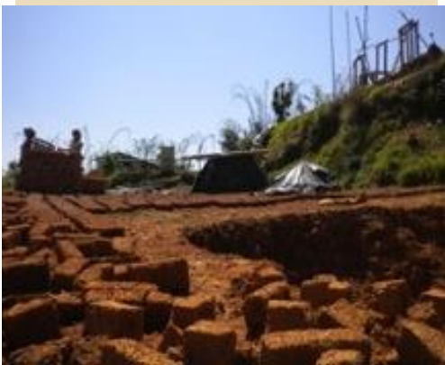
Mud bricks drying in the sun for construction in Okhaldhunga
