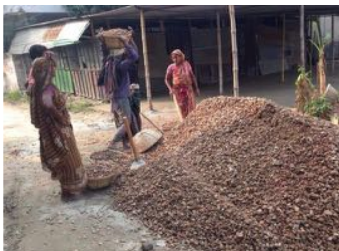
Women working in construction site.
