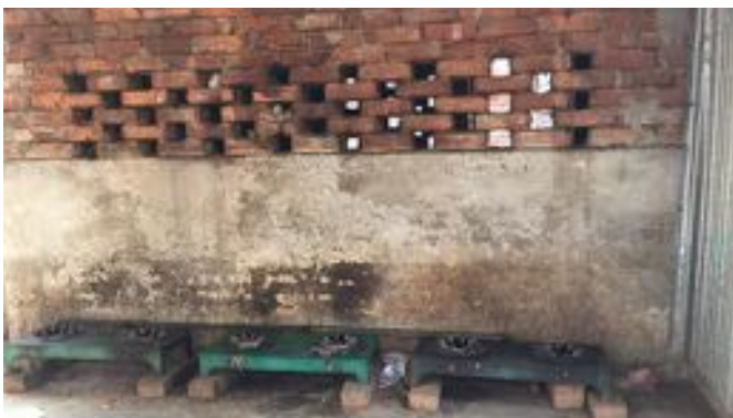
Pipeline gas supply is usually sufficient in the early mornings.
