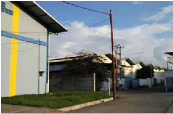
Typical factories in Tangerang Urban Industrial, but those which are said to be good places to work have extensive document requirements from applicants
