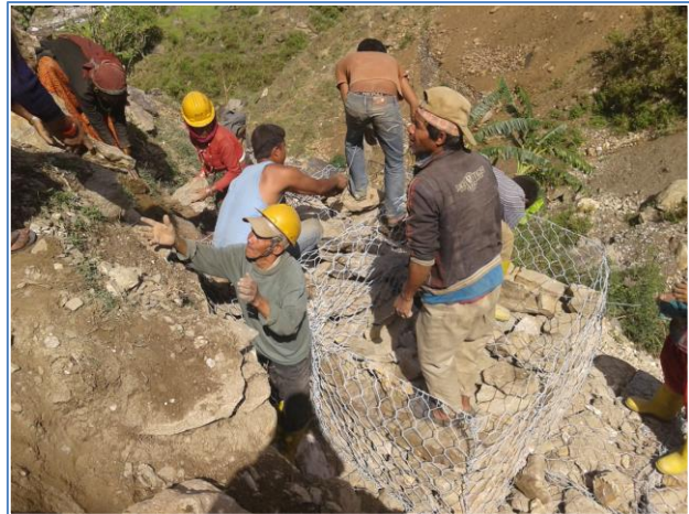
Men working to build gabion wires and retention walls
