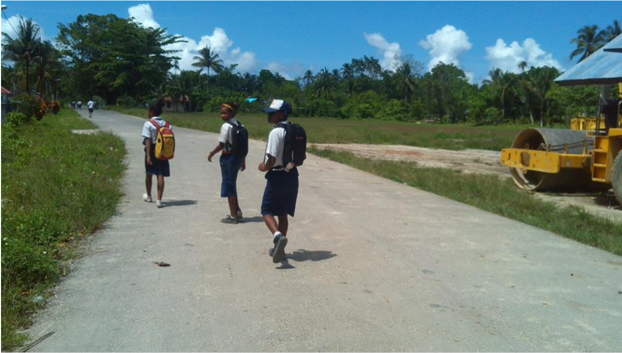
New road construction has just finished
