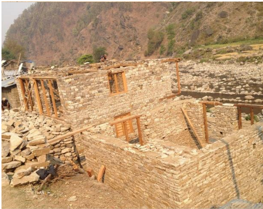
lots of new construction in Accham study location....
