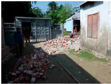
Useful construction has taken place in many government primary schools during PEDP2, but there is little attention to health and safety.
