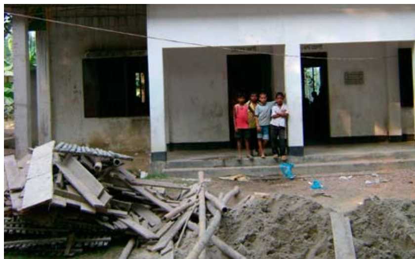
Building work on the primary school is causing considerable disturbance
